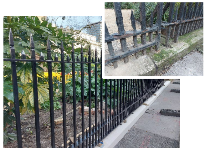
Railings before (top) and after repair
