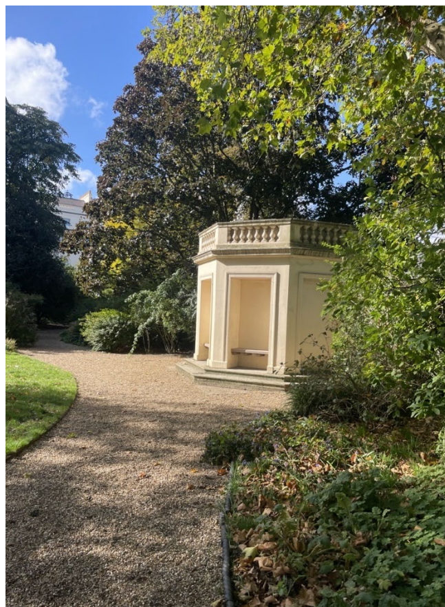
Vent shaft in Park Crescent
